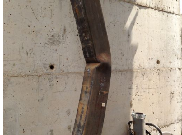
Figure 14. Local Buckling of HSS Element after HSS Test 2
