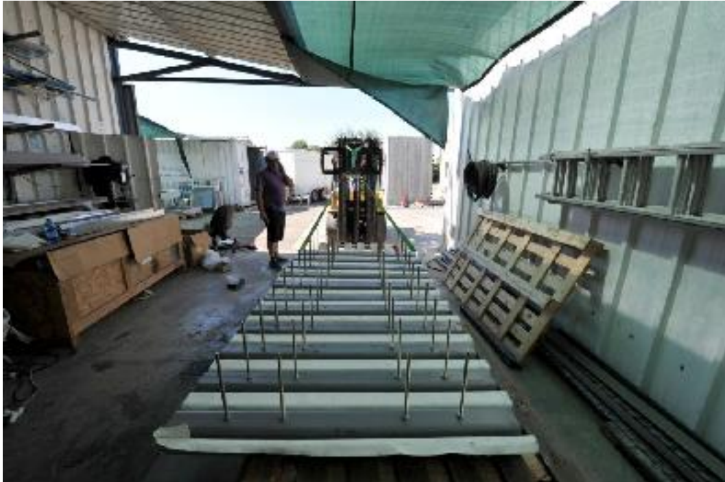
Figure 24 Assembly of the Cladding for HSS Target
