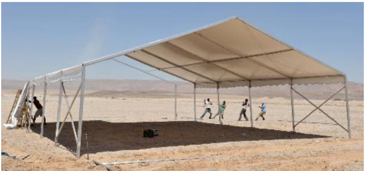
Figure 12 Tent being erected on-site
