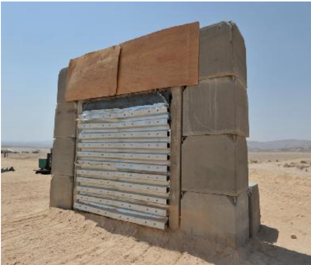
Figure 43 HSS Target Repaired Prior to Second Test
