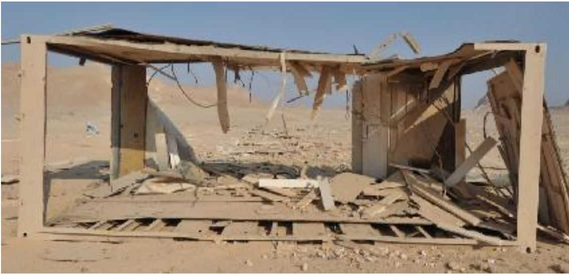
Figure 46 Modified Steel Framed Sea Container Office Following Test 2
