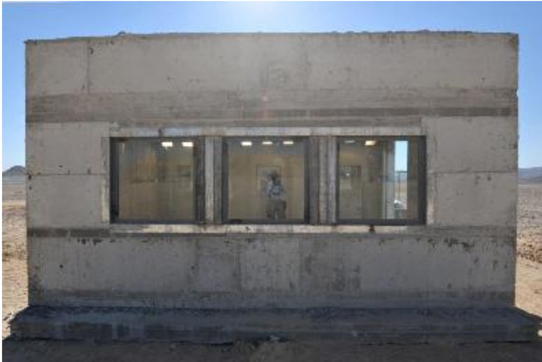
Figure 30 GFPM Target Prior to First Test
