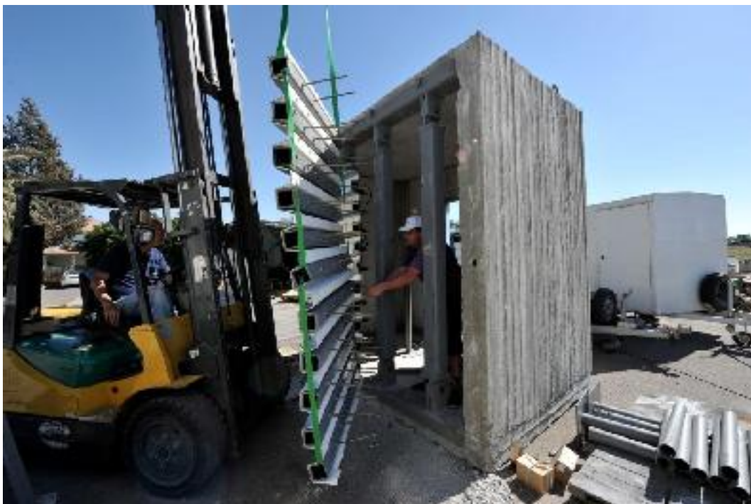
Figure 25 Installation of Cladding on HSS Target
