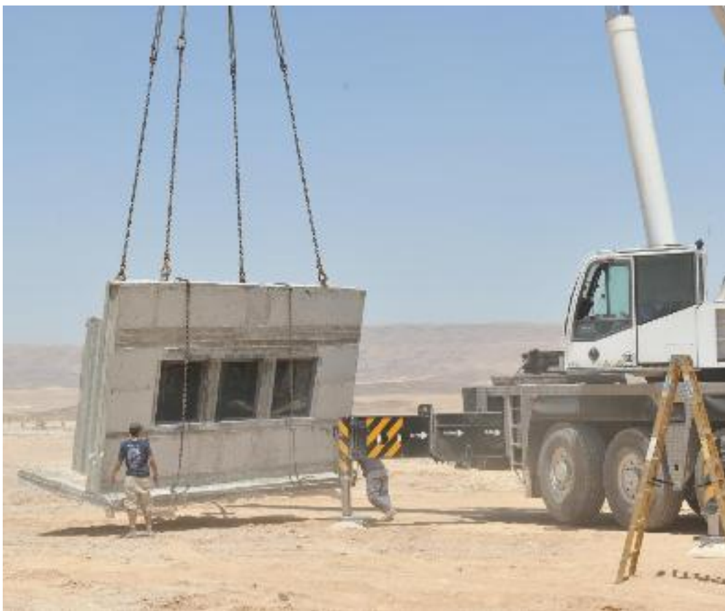
Figure 29 Lifting GFPM Target into Arena
