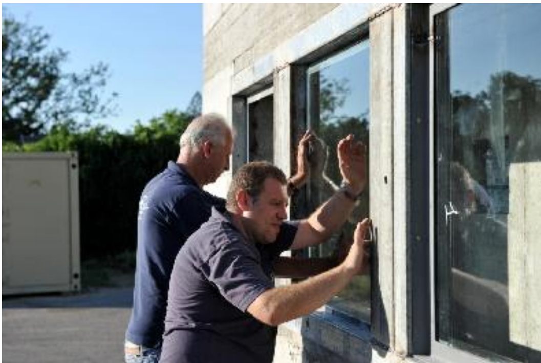
Figure 28 Glass Panes and Supports Being Installed into GFPM Target
