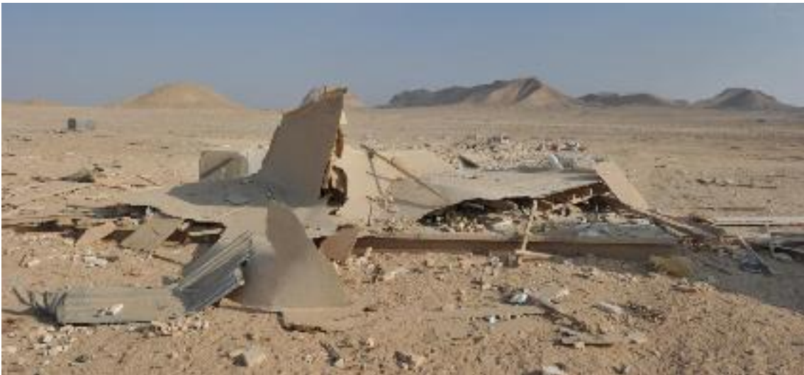
Figure 47 Site Office Following Test 2
