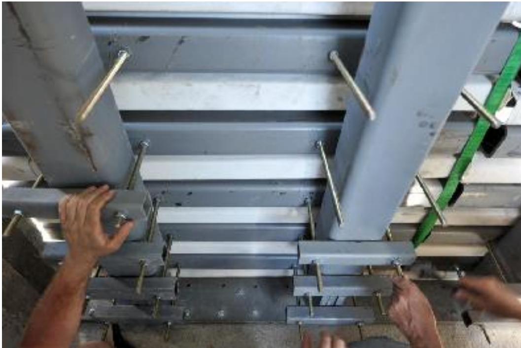
Figure 26 Tightening of Cladding Supports for HSS Target
