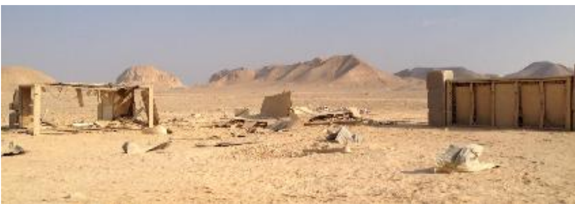
Figure 48 EDC Target, Shipping Container Office, and Site Office after Test 2
