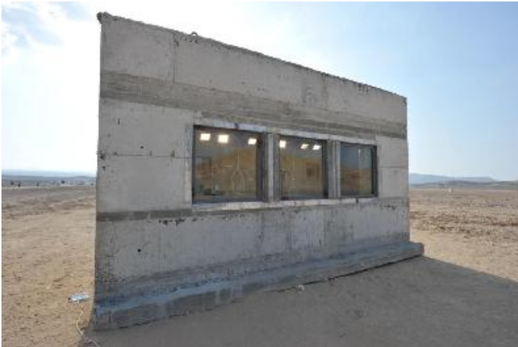
Figure 42 GFPM Target Prior to Test 2 with Broken Window Replaced
