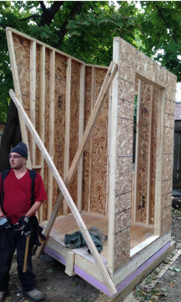
Wood Frame Construction
