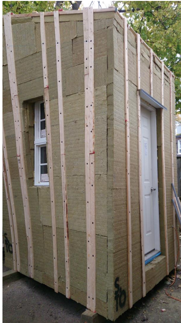
Wood Furring for Siding
