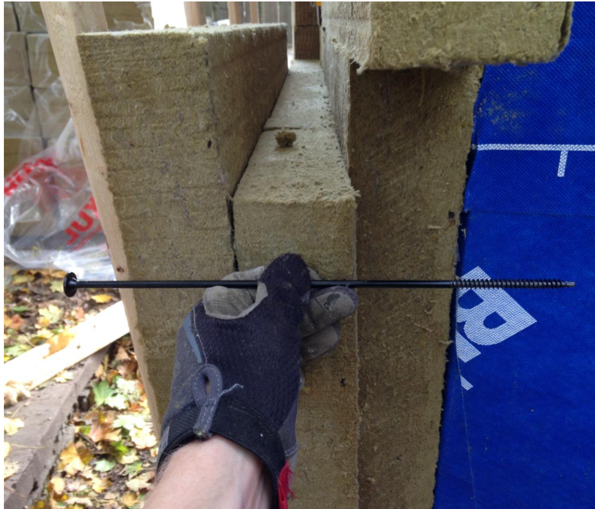
Long 12" TruFast SIP screws fastened through furring and insulation to stud wall
