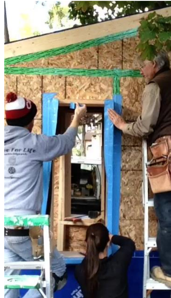
Weather and air sealing at window buck extension
