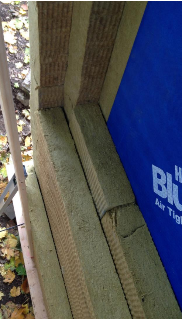
Layering insulation, 3" lapped seams
