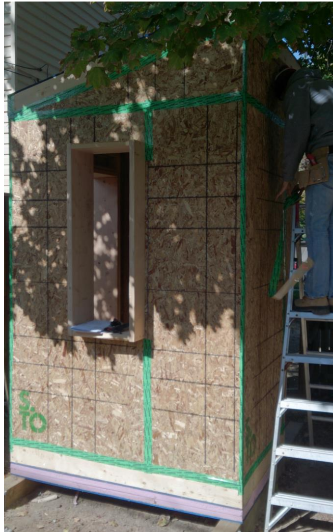
SIGA tape on sheathing – continuous air barrier, OSB vapour control
