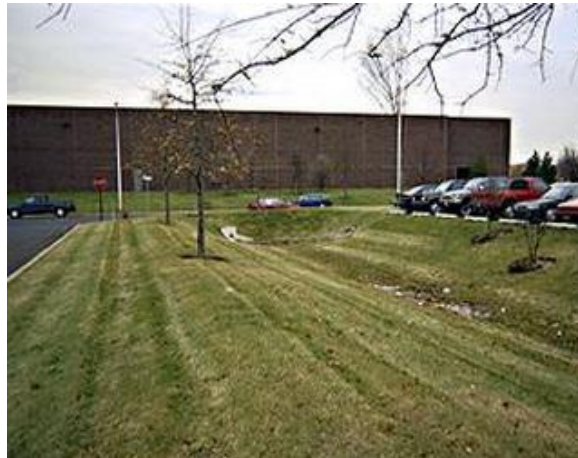
Enhanced Grass Swale
